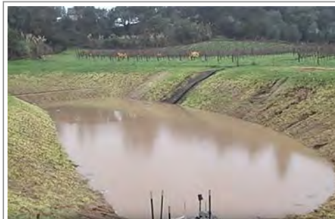
Groundwater recharge basins collect excess runoff during heavy rains and allow the water to infiltrate into the soil and replenish the groundwater supply.
